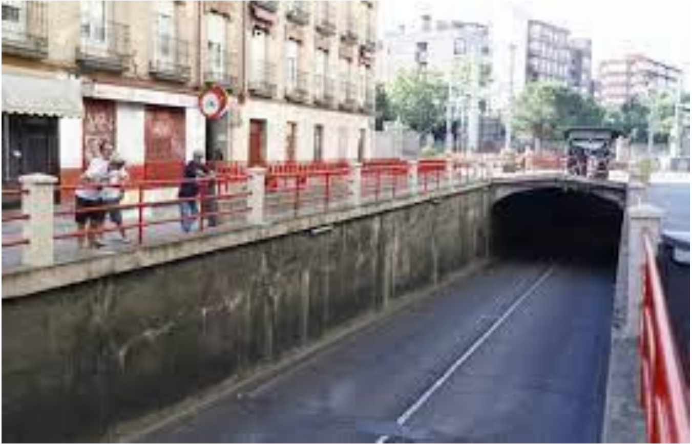
Figure 28. Car tunnel in Valladolid.
