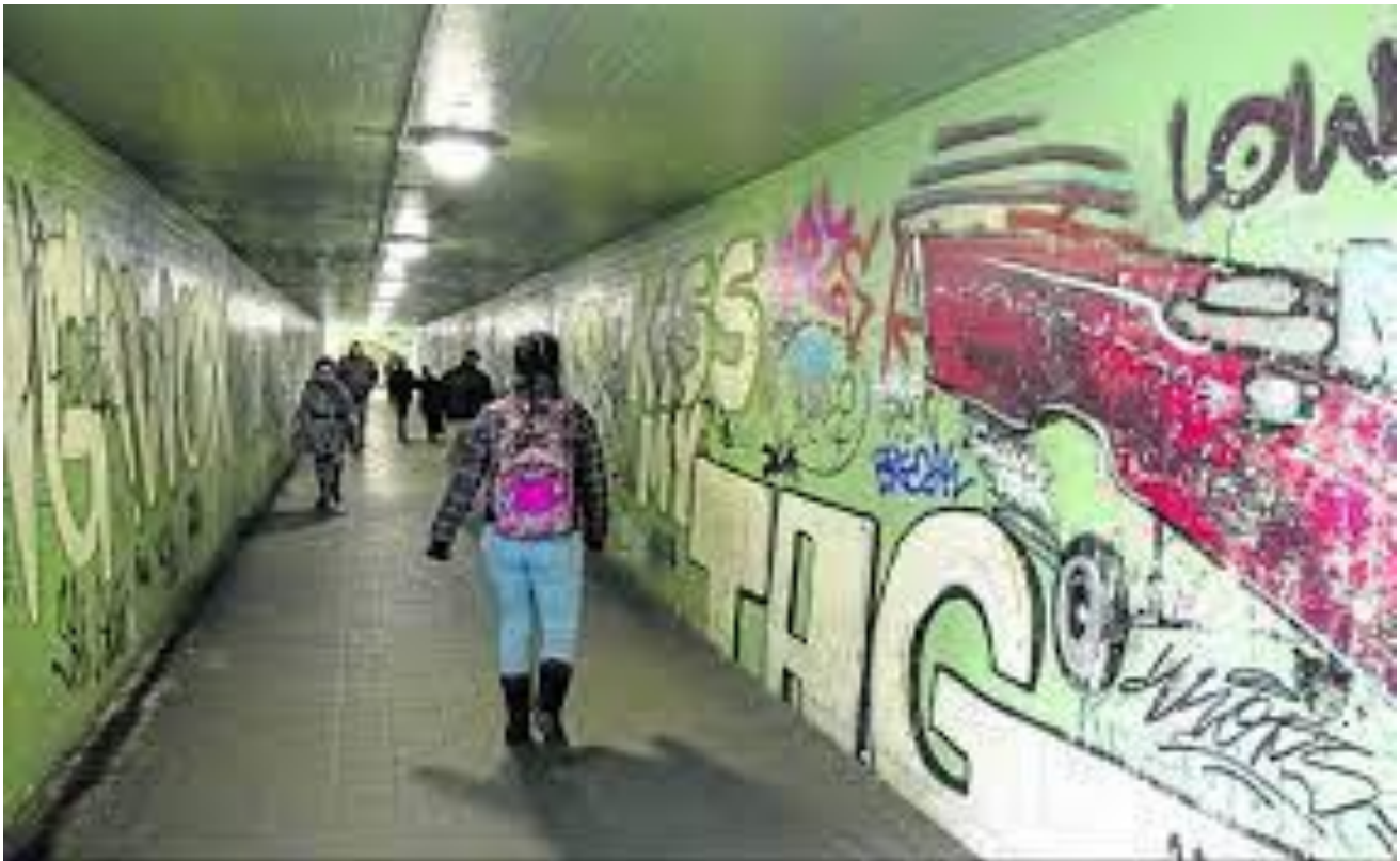
Figure 27. Pedestrian tunnel in Valladolid.
