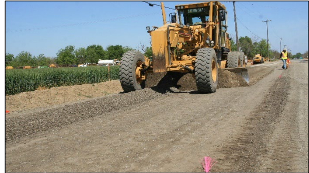
Figure 6.5: Adding new layer for structural improvement prior to recycling.
