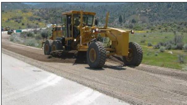
Figure 6.99: Shaping and final leveling with a grader on FDR projects.
