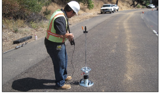
Figure 6.116: Checking stiffness reduction with a light weight deflectometer.
