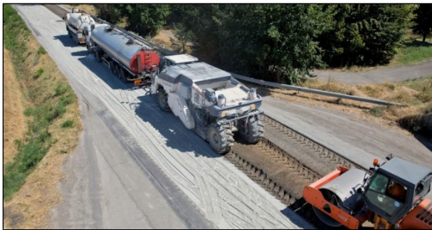
Figure 6.8: Wheel-driven FDR recycling train.
