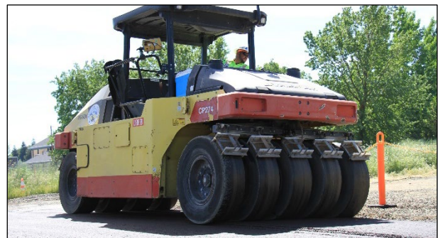
Figure 6.14: Pneumatic-tired roller on a PDR layer.
