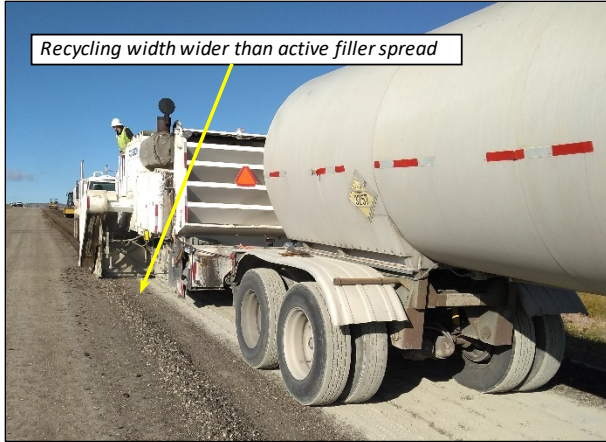
Figure 6.67: Spreading active filler in a strip that is narrower than the recycler (FDR).
