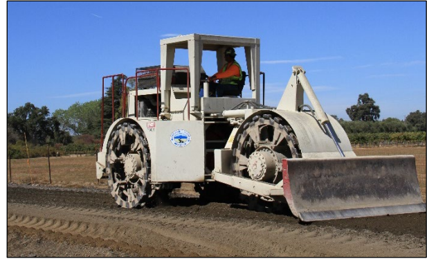
Figure 6.16: Segmented padfoot roller on an FDR-C layer.
