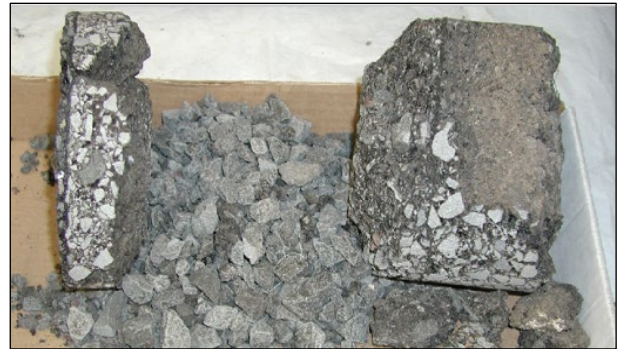
Figure 2.48: Stripped asphalt concrete layer.
