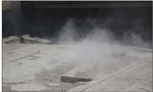
Figure 6.65: Pan after spreader has passed on an FDR-C project (4% stabilizer).
