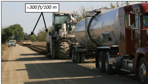
Figure 6.97: Typical maximum distance of padfoot roller behind recycling train (FDR).
