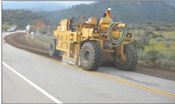
Figure 6.55: Prepulverization on an FDR project.
