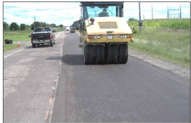
Figure 6.85: Primary compaction with pneumatic-tired roller on a PDR project.
