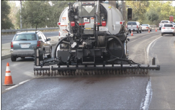
Figure 6.108: Curing seal application on a PDR project.
