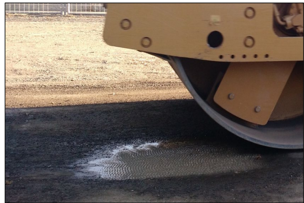
Figure 6.114: Close-up view of microcracking showing vibrations applied to road surface.
