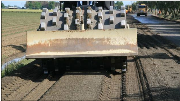
Figure 6.91: First padfoot roller pass on an FDR project.
