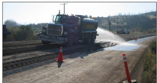
Figure 6.76: Separate water application behind recycler (FDR).
