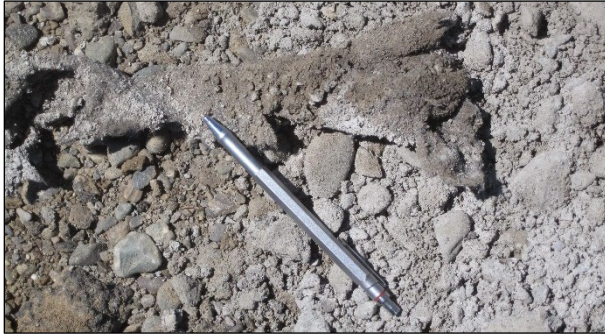
Figure 6.36: Fabric behind the recycler on an FDR project.
