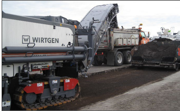
Figure 6.81: Removing excess material on a PDR project.
