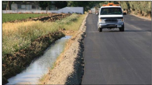
Figure 2.9: Example use of side drain to move irrigation water.
