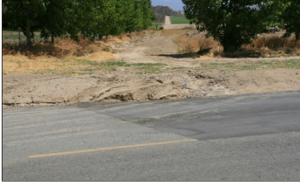
Figure 2.2: Example road below natural ground level.
