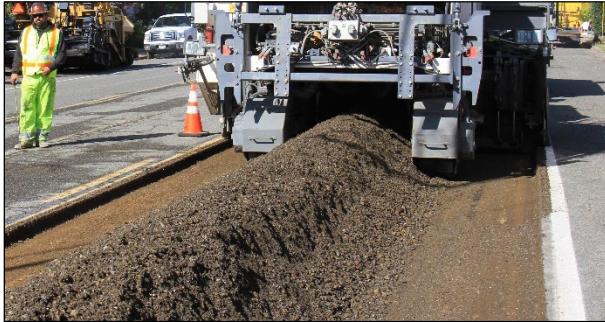
Figure 6.32: Good gradation and consistency behind the recycler on a PDR project.
