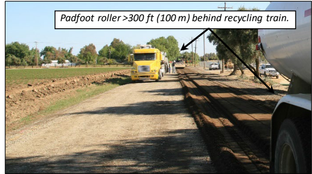
Figure 6.96: Primary compactor too far behind recycling train (FDR).
