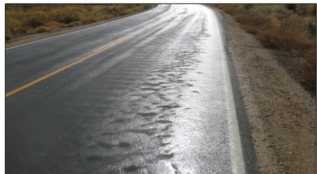
Figure 6.100: Effect of padfoot impressions on overlay smoothness (FDR).
