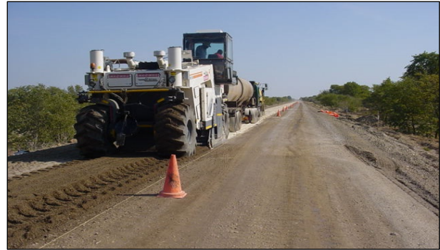
Figure 6.59: String line for direction and overlap guides for the recycling train (FDR).
