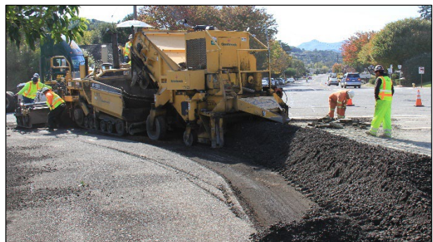
Figure 6.80: PDR project with pickup machine feeding the paver.
