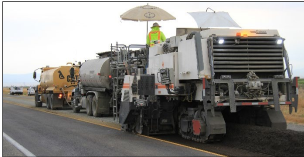
Figure 1.2: Partial-depth recycling train (single unit).
