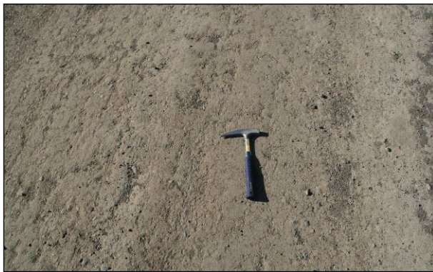
Figure 6.121: Acceptable surface prior to tack coat application.
