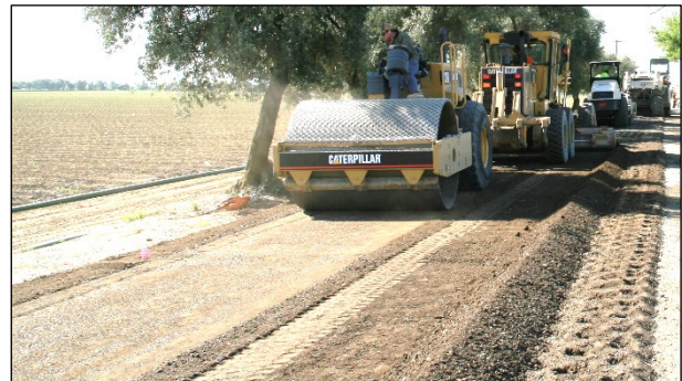
Figure 6.98: Final leveling and compaction interfering with primary compaction (FDR).
