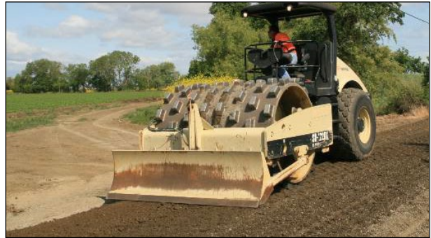
Figure 6.92: Using the blade to drag material into padfoot impressions (FDR).
