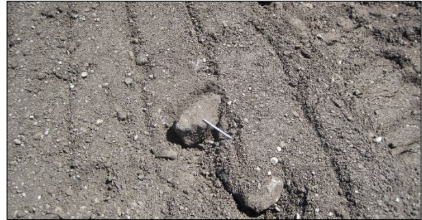
Figure 6.33: Oversize material behind the recycler on an FDR project.
