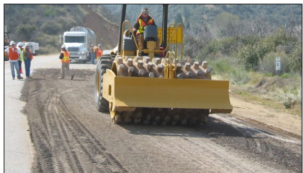
Figure 6.94: Padfoot impressions after multiple roller passes (FDR).
