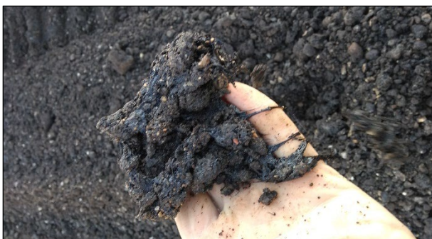
Figure 6.44: Poorly dispersed asphalt recycling agent (nozzle problem).
