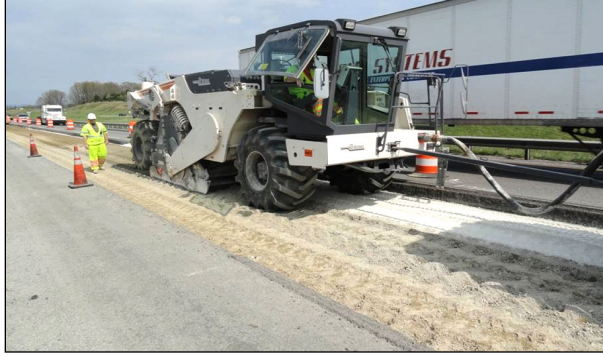
Figure 3.4: Stabilizing lower layers/subgrade prior to placing a CCPR layer.
