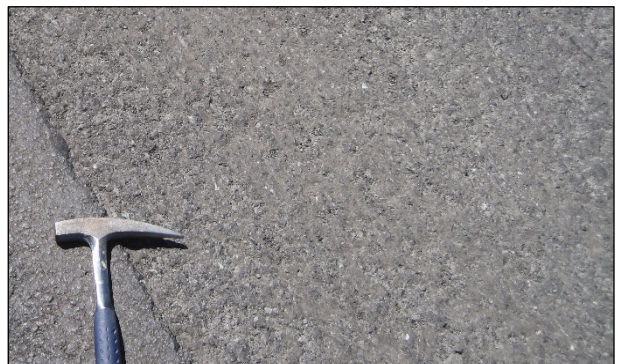
Figure 6.119: PDR layer milled for smoothness prior to placing asphalt concrete surface.
