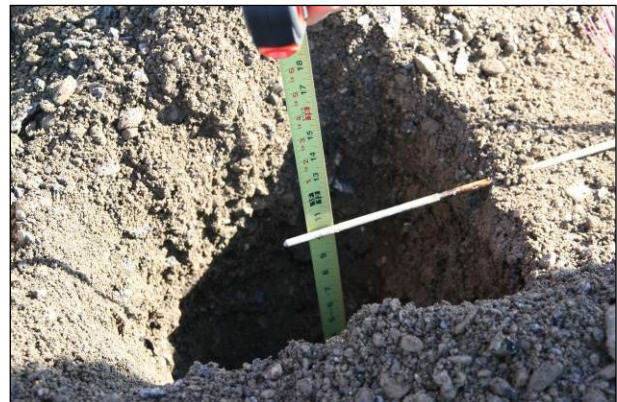
Figure 6.28: Checking recycling depth in a hole on an FDR project.
