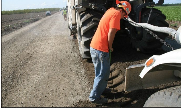
Figure 6.29: Checking recycling depth using a T-bar on an FDR project.
