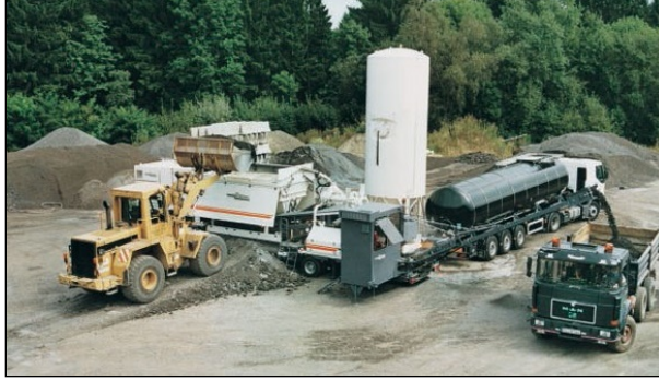
Figure 1.6: Central plant recycling.
