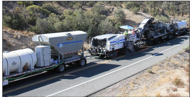
Figure 1.3: Partial-depth recycling train (multi-unit).
