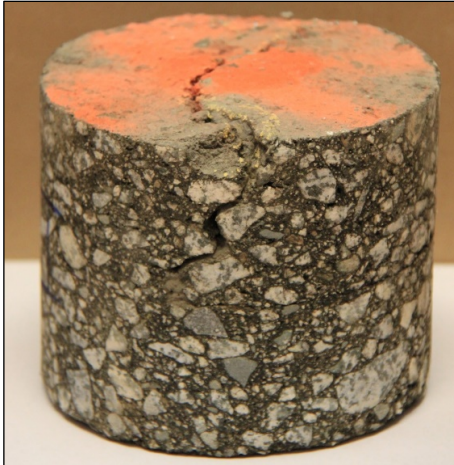
Figure 2.41: Top-down thermal crack.
