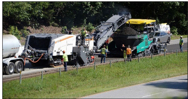
Figure 6.9: Track-driven recycling train for PDR and FDR (down to 12 in. [300 mm]).
