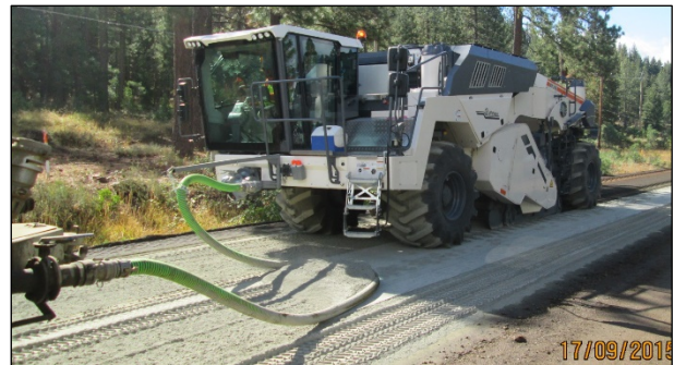
Figure 6.18: Recycler with no push bar and hose dragging cement stabilizer (FDR-C).
