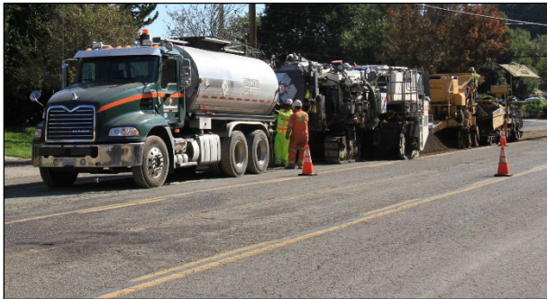
Figure 6.6: Single-unit PDR recycling train.
