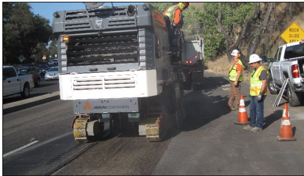
Figure 6.2: Premilling to maintain crossfall prior to PDR.
