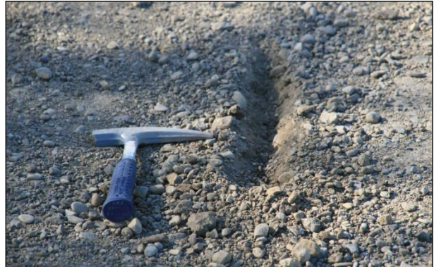
Figure 6.101: Segregation after excessive movement of material with a grader (FDR).
