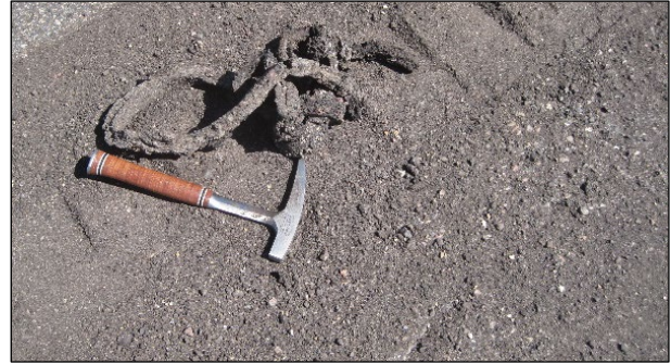
Figure 6.37: Crack seal behind the recycler on a PDR project.
