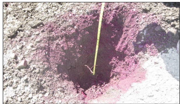
Figure 6.47: Checking cement mixing depth on an FDR-C project (note crimson color).
