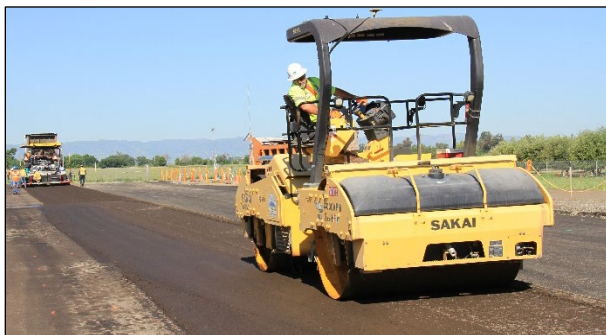
Figure 6.13: Steel breakdown roller on a PDR layer.
