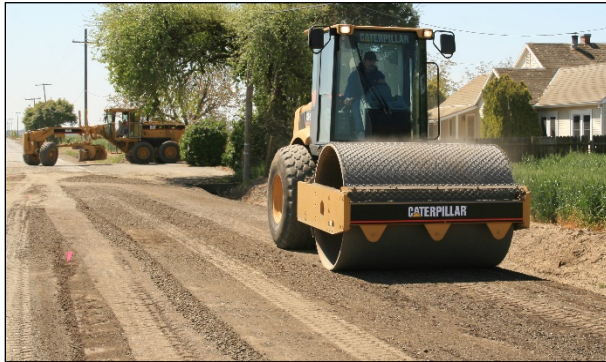
Figure 6.103: Intermediate rolling on FDR layer with single drum steel roller.
