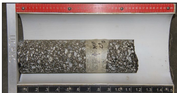
Figure 2.49: Core from digout showing 1.15-ft thick asphalt concrete layer.
