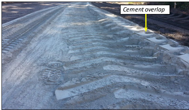
Figure 6.71: Overlap of cement spread on an FDR-C project (double application).
