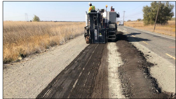
Figure 6.3: Premilling to include shoulders in a PDR project.
