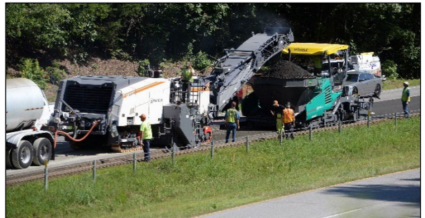
Figure 1.5: Full-depth recycling train (track).
