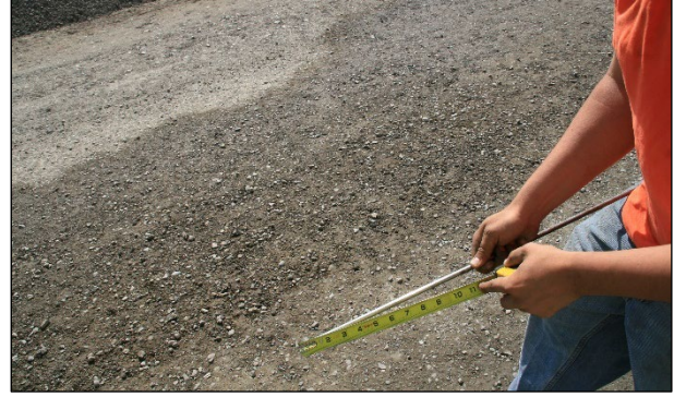
Figure 6.30: Measuring recycling depth on the T-bar (FDR).
