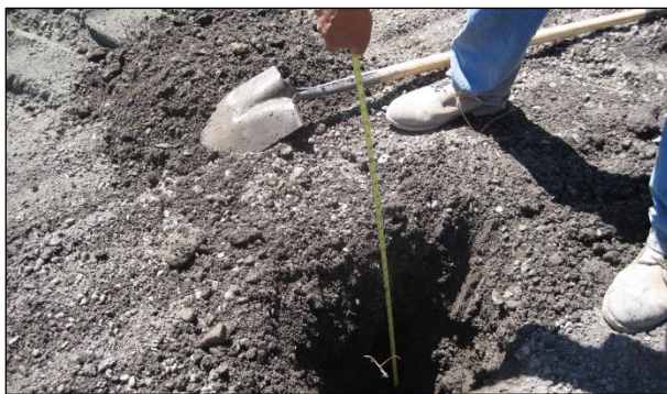
Figure 6.46: Checking recycling depth on an FDR-C project.
