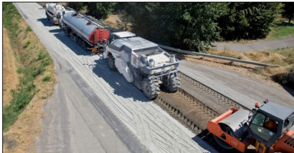
Figure 1.4: Full-depth recycling train (wheel).
