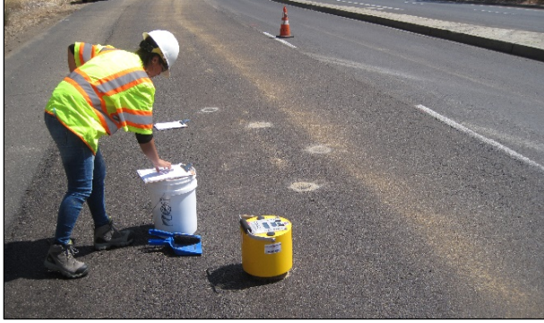
Figure 6.115: Checking stiffness reduction with a soil stiffness gauge.
