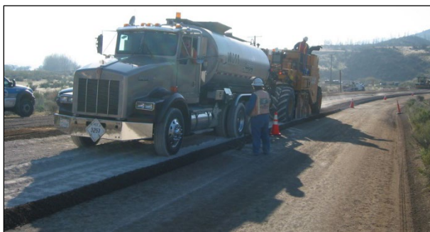
Figure 6.75: FDR-FA recycling train with no water tanker.
