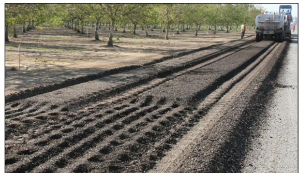
Figure 6.83: Partial compaction by recycling train wheels on an FDR project.
