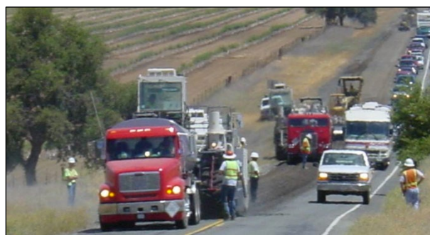
Figure 6.1: Pilot car traffic control on FDR project.
