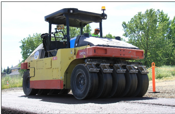
Figure 6.85: Primary compaction with pneumatic-tired roller on a PDR project.
