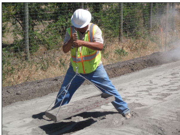
Figure 6.66: Weighing a calibration pan on an FDR-C project.
