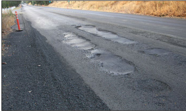
Figure 6.120: Patched distressed areas prior to surfacing.
