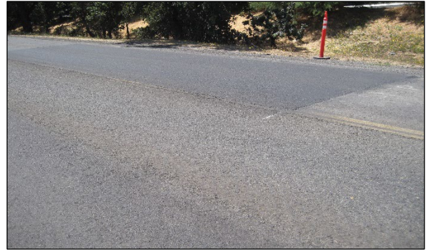
Figure 6.120: Patched distressed areas prior to surfacing.
