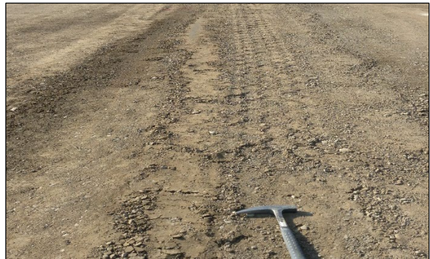
Figure 6.102: Delamination after blading thin lifts of material during grading (FDR).
