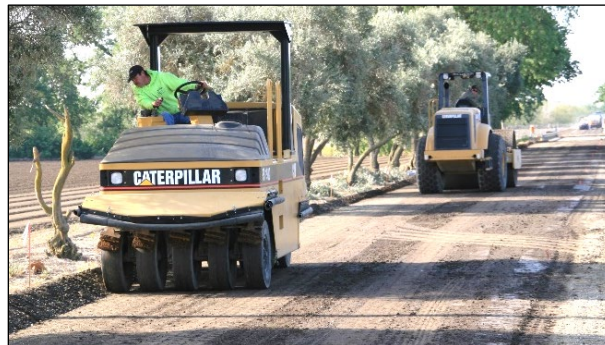
Figure 6.105: Intermediate rolling on FDR layer with steel-drum and pneumatic-tired rollers.
