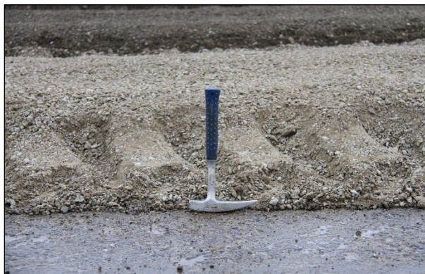
Figure 6.56: Bulking of material after prepulverization to a depth of 12 in. (300 mm).
