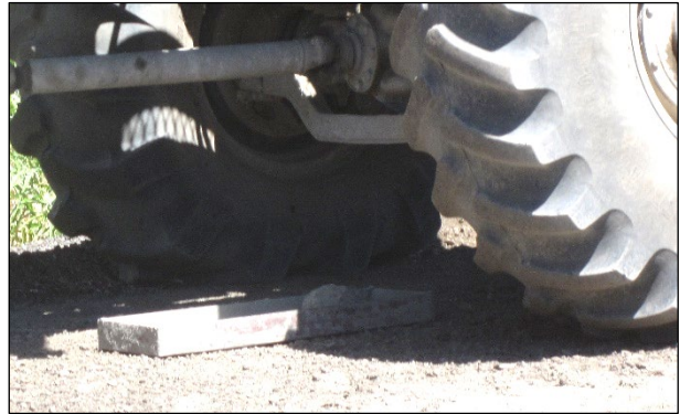
Figure 6.63: Spreader passing over pan on a prepulverized FDR-C project.
