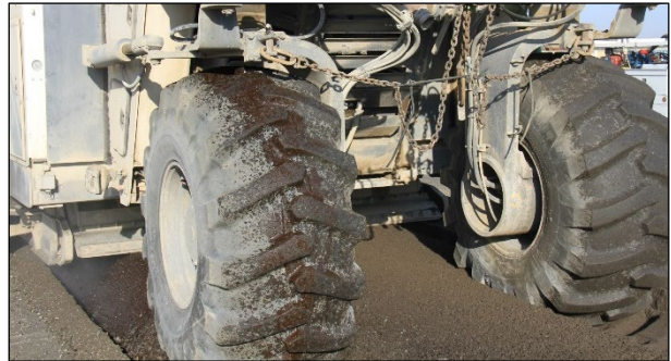
Figure 6.40: Effect of problem nozzles on an FDR-EA project.
