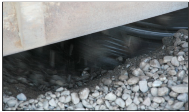
Figure 6.24: Localized segregation caused by idling recycler drum (FDR).
