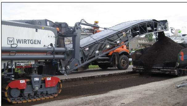
Figure 6.79: PDR project with belt feed into paver.
