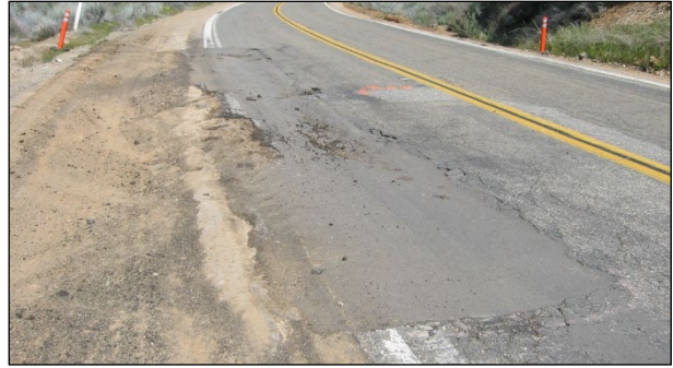
Figure 2.18: Example top-down distresses: Edgebreak.
