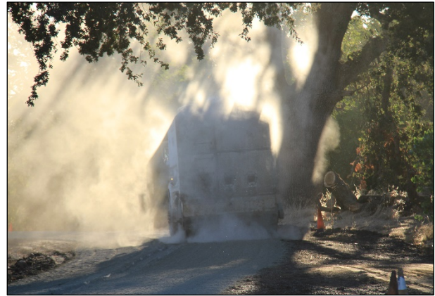
Figure 6.74: Loss of active filler/stabilizer during windy conditions.
