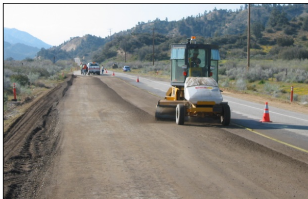
Figure 6.107: Light brooming prior to curing seal application on an FDR project.
