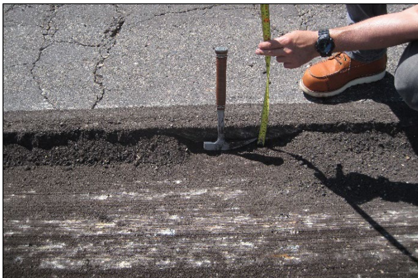
Figure 6.27: Checking recycling depth on a PDR project.
