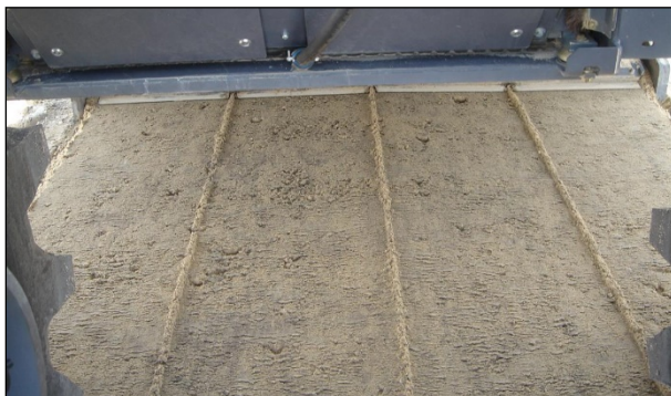
Figure 6.82: Material behind mixing chamber on FDR project with wheel-driven recycler.
