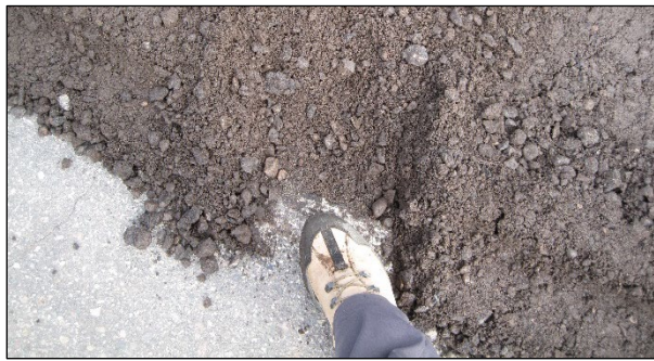
Figure 6.38: Clearing marks in overflow material to guide roller operators.
