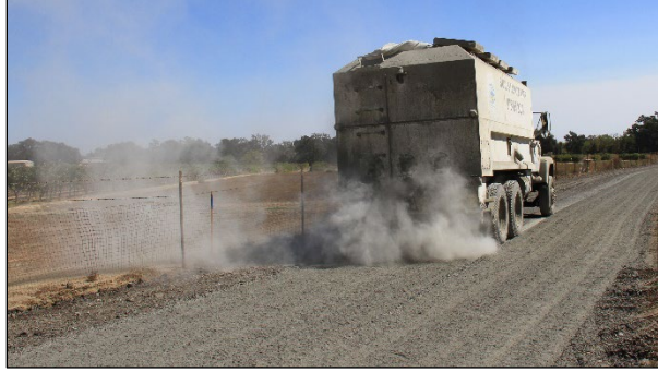
Figure 6.12: Active filler/stabilizer spreader.
