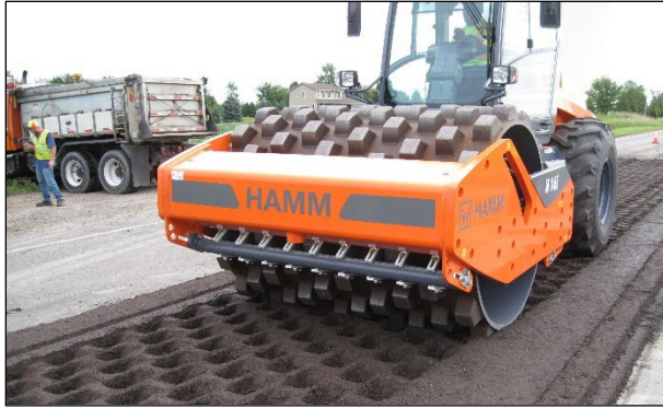
Figure 6.15: Vibratory padfoot roller on an FDR-FA layer.
