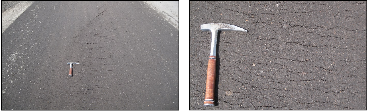
Figure 6.89: Shearing after completion of primary compaction on a PDR project.
