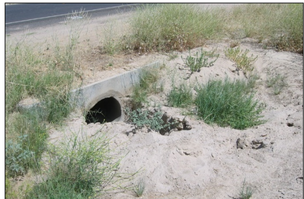
Figure 6.124: Soil blocking a culvert after completing an FDR project.
