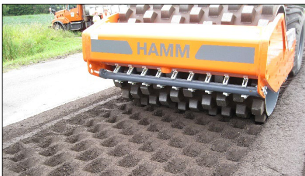
Figure 6.93: Padfoot impressions after first roller passes (FDR).
