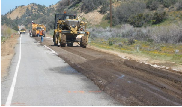
Figure 6.77: Water application between recycler and primary compaction roller (FDR).
