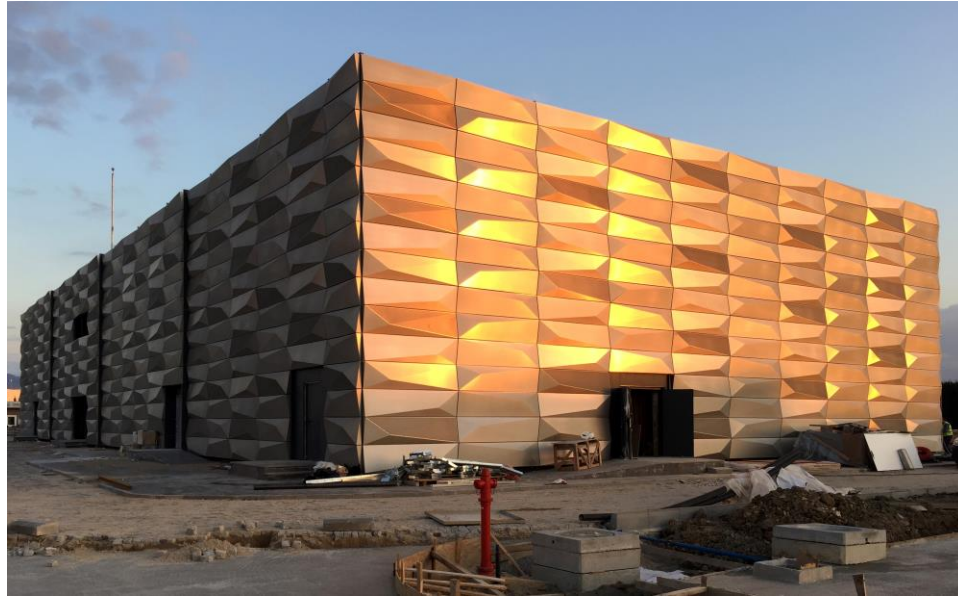
Fig. 9. Back of metal façade changing with daylight. Sakarya Industrial Zone Headquarters and Conference Hall , Sakarya, Turkey, under construction, completion September 2016. Photo credit: BINAA.
