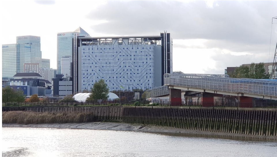
Figure 4. Telehouse North Two
